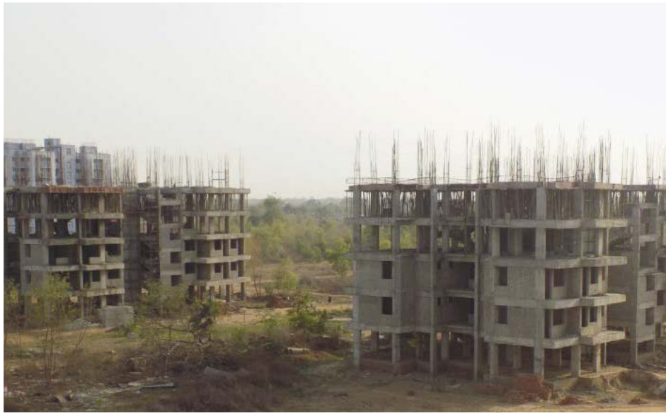
C type Quarters (Capacity: 56 units) 40% complete(RCC of 5 th floor is in progress)
