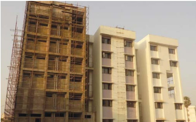
Girls Hostel (Capacity: 200) 90% complete (Painting, fittings and fixing in progress)
